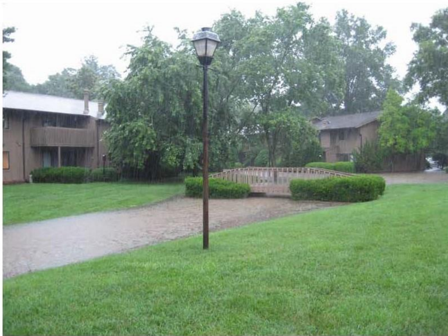
Stream running under the walkway bridge in front of Building 1800...
