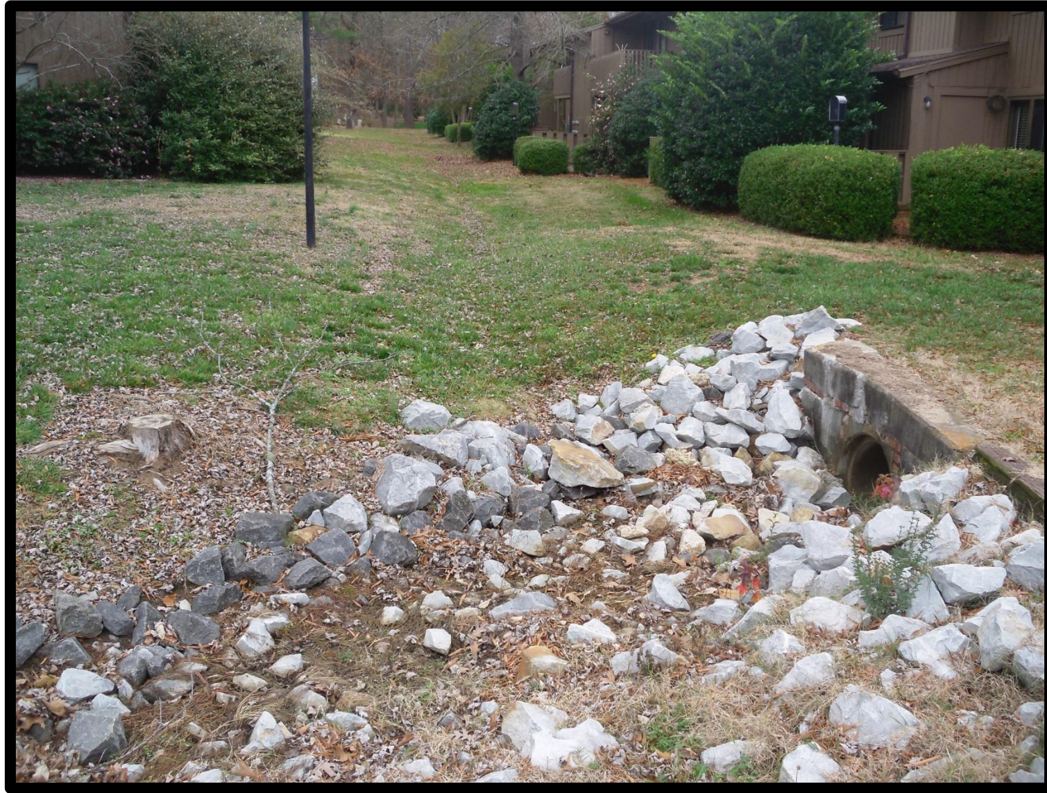
Drainage Alignment Behind Buildings
