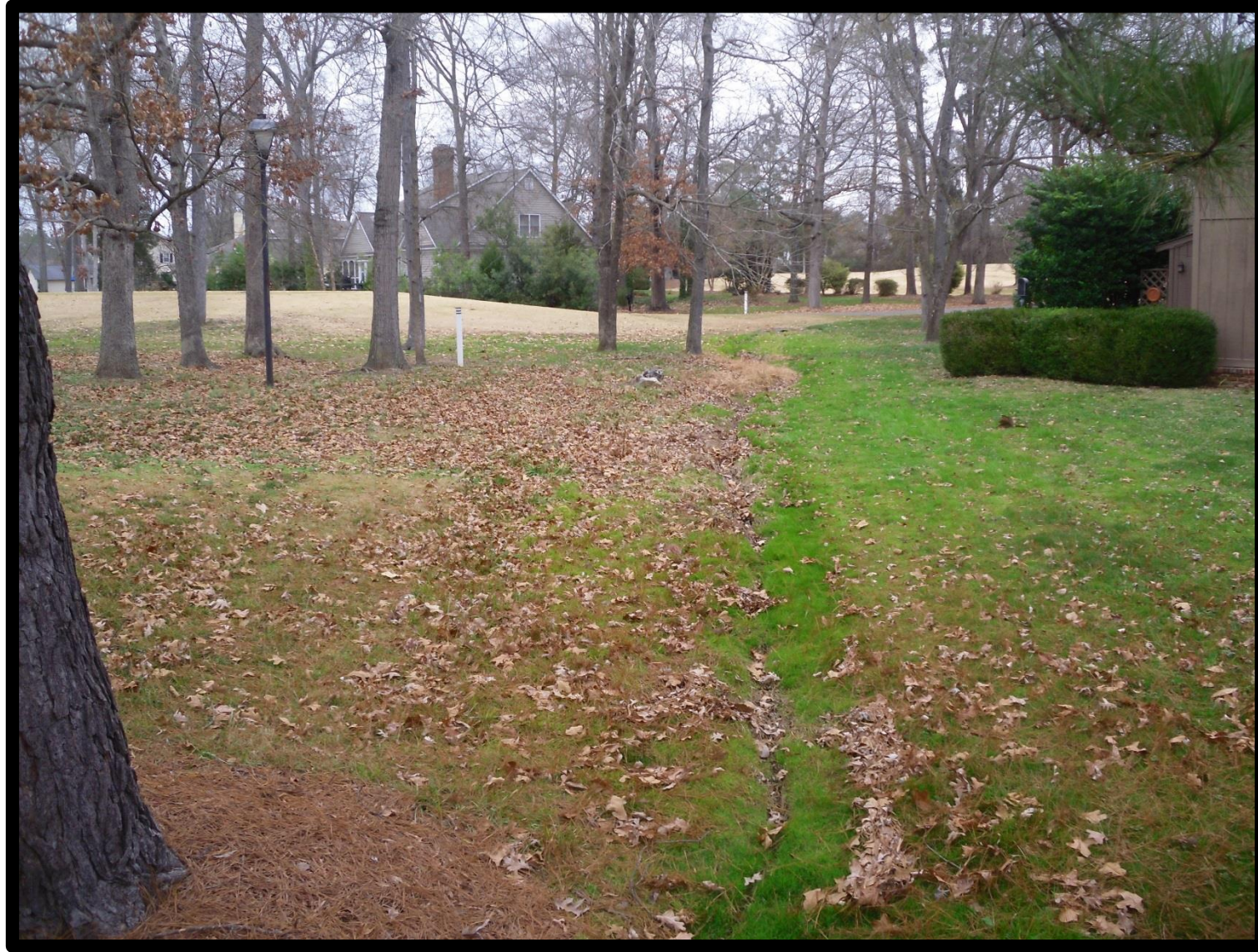
Drainage Alignment at First Junction Box
