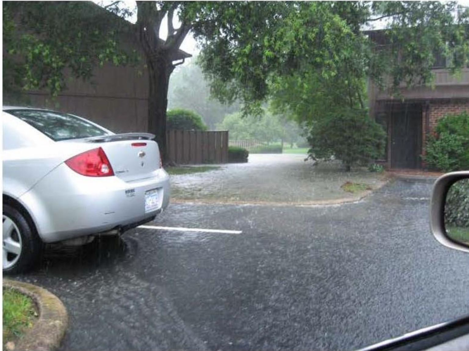
Stream overflowing into parking lot between Buildings 1400 & 1500 ...
