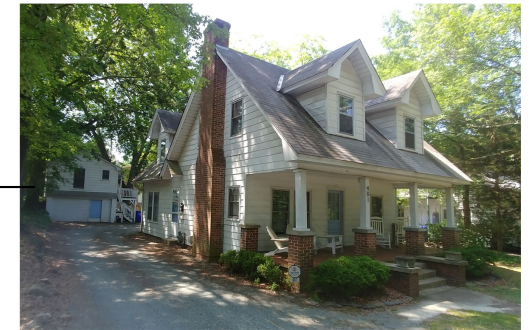
401 W Patterson - 1.75 story Lot: .23 ac - Floor Area: 2,065 sf. - Floor Ratio: .206 Porch Eave - 10'-8" Dormer Eave - 21'-6" Ridge - 27'-10"
