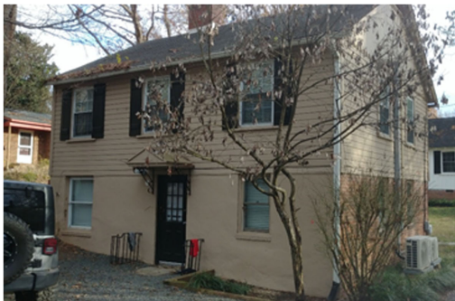
413 W Patterson - 2 story Lot: .14 ac - Floor Area: 1,344 sf - Ratio: .22 Roof Eave - 16'-10" Ridge - 23'-8"
