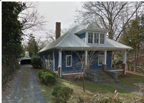
409 W Patterson - 1.5 story Lot: .27 ac - Floor Area: 1,830 sf - Floor Ratio: .16 Porch Eave - 14'-0" Dormer Eave - 18'-0"
