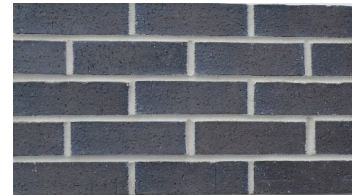
BRICK MASONRY VENEER
