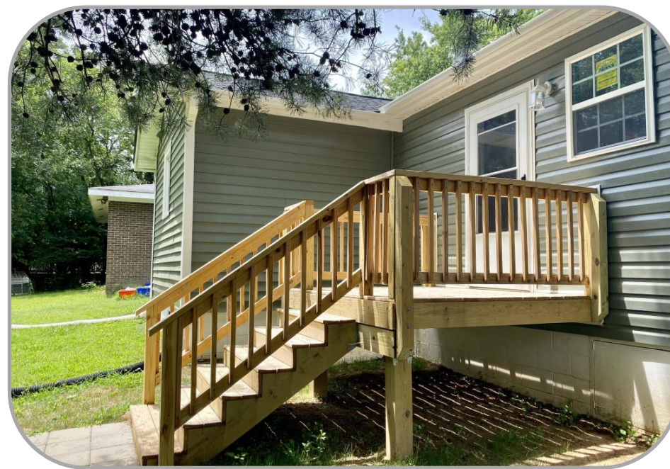
Home Repairs & Rehabilitation
