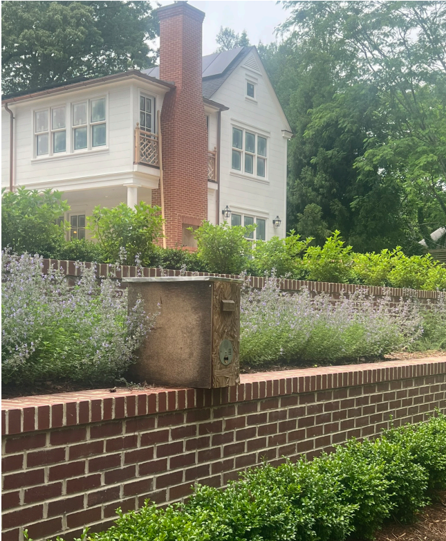
EXISTING BRICK RETAINING WALL
