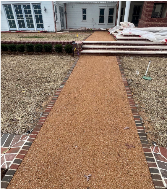
EXISTING C.H. GRIT PATHWAY WITH BRICK CURBING
