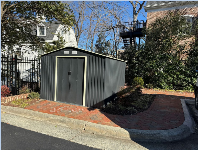
Existing Metal Shed
