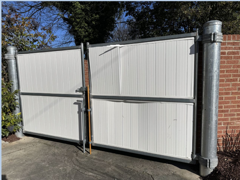
Existing Dumpster Panels
