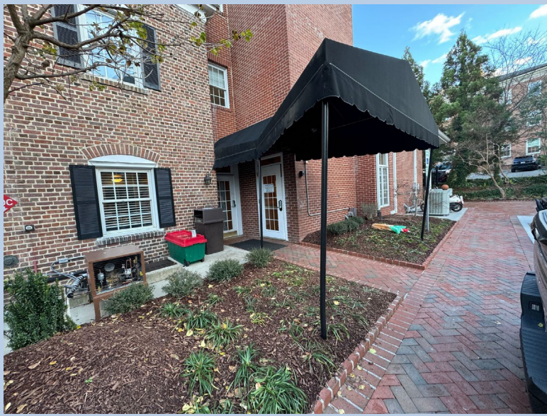
Existing Rear Entrance Canopy
